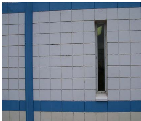
Exterior view of the rear window of the Ward’s room
