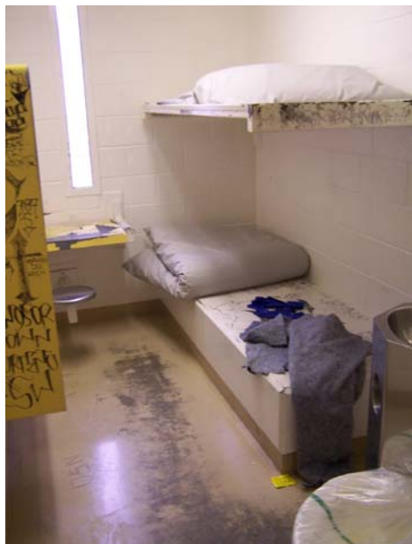
Picture taken from doorway, looking into the Ward’s room
